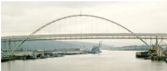
Figure 9 Old bridge over the bay.
