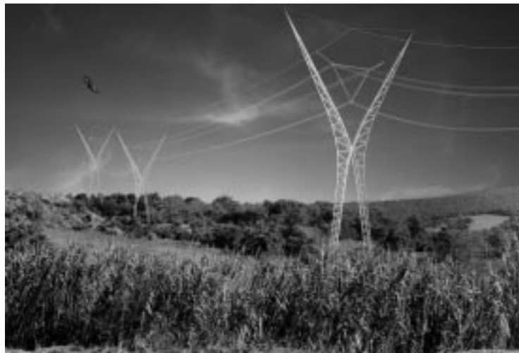
Fig. 11: A different style of masts for high-voltage power cables
